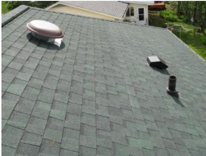
North side of roof.
